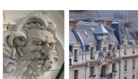
Ilot Terreaux - Mauborget, Lausanne.
